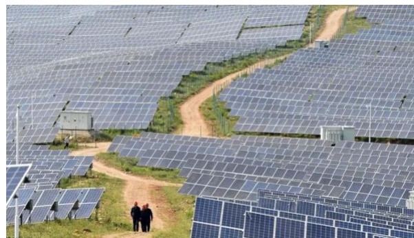
Figure 1: Workers inspect a solar power plant in a Chinese province. 33
